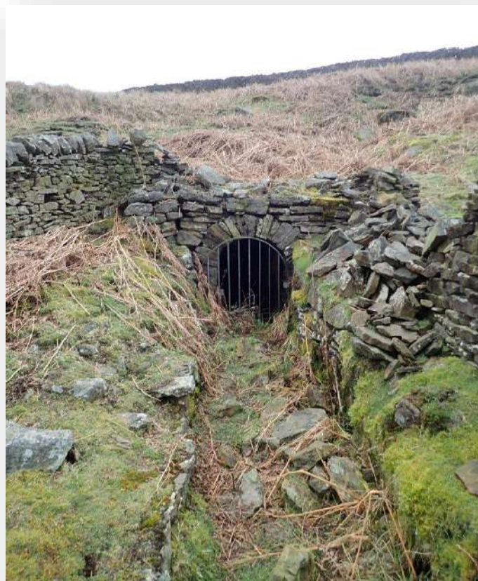
Figure 8 Example of Stone Arched Adit
