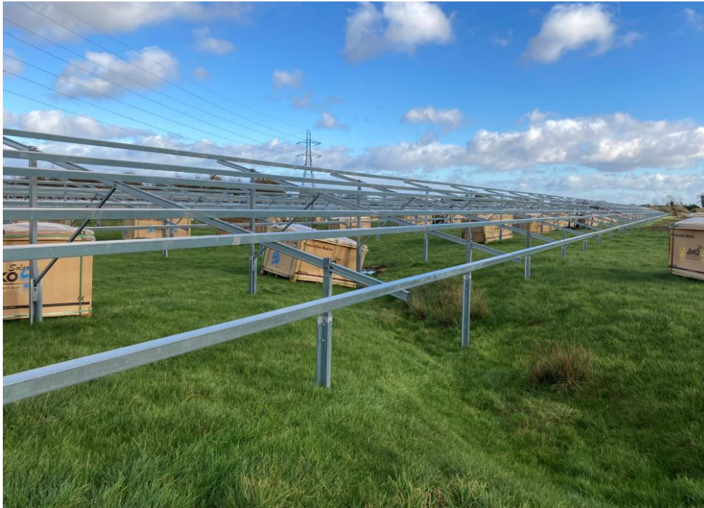
Photograph 1: Illustrative photo showing solar frame installation
