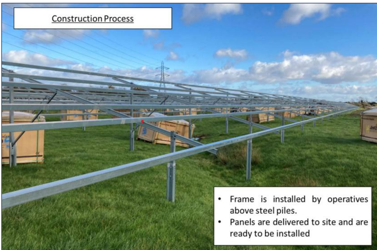
Figure 15 Photograph showing the framework system prior to bolting on the panels.
