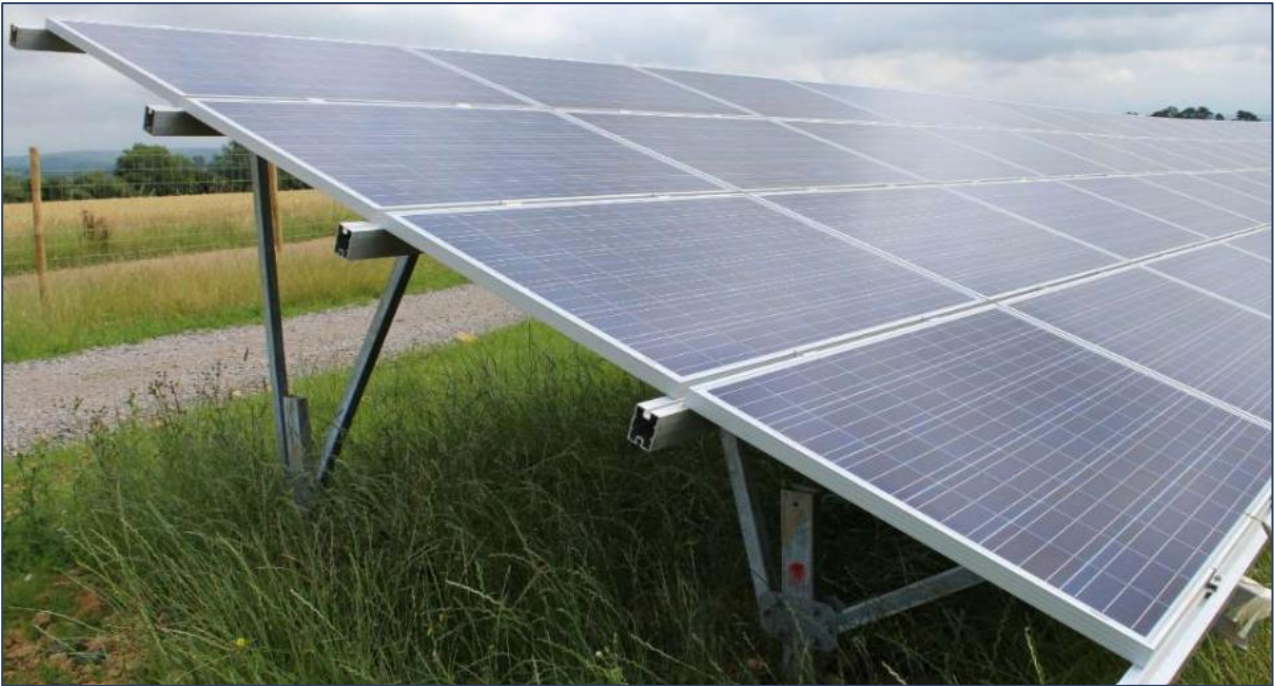
Figure 14 Photograph showing the arrays with standard gaps between panels to allow rainwater to flow through and disperse the run off.
