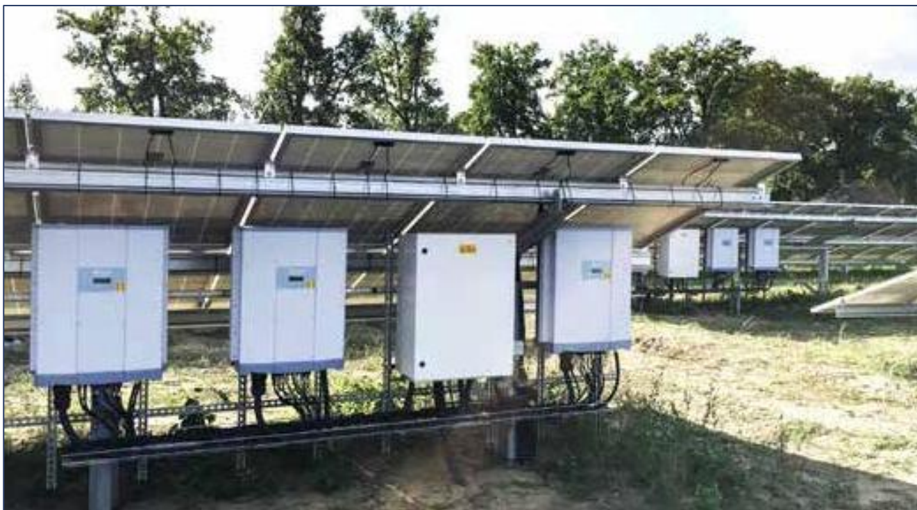
Figure 17 Photograph of inverters at the end of the 'string' of panels
